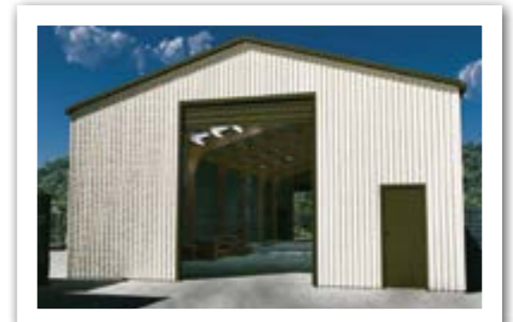
Laminated Veneer Lumber (LVL) timber portal frames used for a Commercial building.
