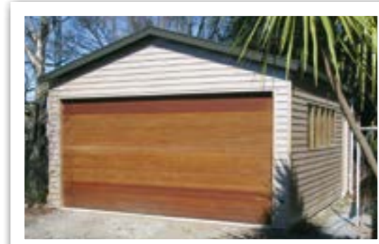
6m x 6m Double Garage featuring a 5.2m cedar sectional door, using Clearcote cladding and Karaka coloured roof and trim.
