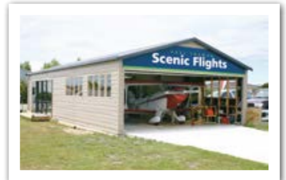
Light aircraft hangar constructed with extra wide sectional door.
