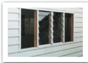
Window louvres provide ventilation.
