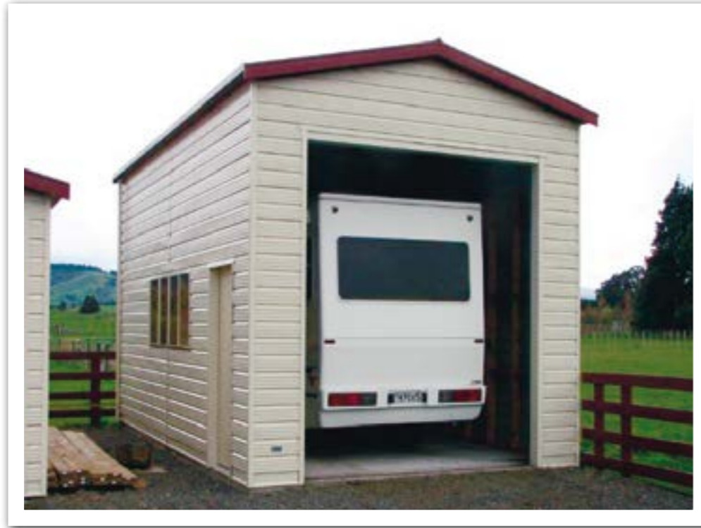
5.4m x 4.2m Garage Workshop with a 3m stud height.
