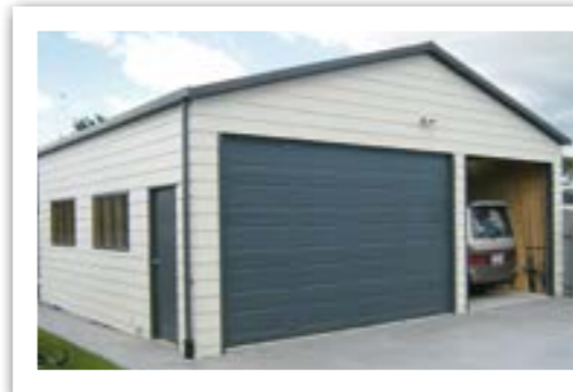
A 10.2m x 9m Garage with Hardiplank cladding, featuring double and single sectional doors.
