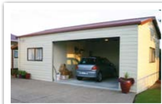
Double Garage with a Sleep Out clad with the popular hidden nail Championboard. Features a separate side door entry to the Sleep Out in addition to the 4.8m main sectional door.
