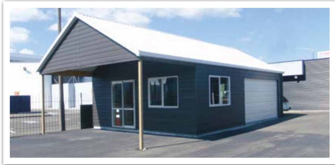
Extended Roofline with New Denim Blue Championboard, featuring Off White coloured roof, door, aluminium joinery and trim.
